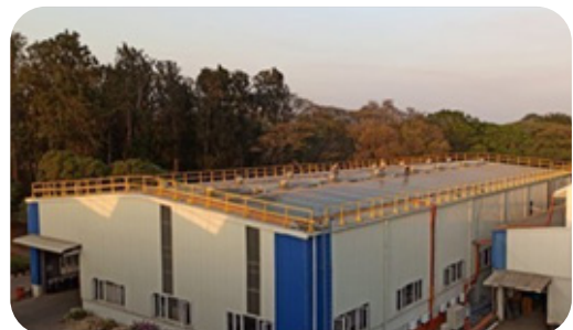
1.14 MW at Hosur unit
