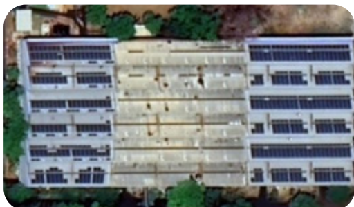
0.35 MW at Krishnapuram unit
